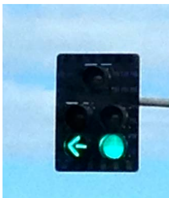
Permissive-protected signals (Doghouse)
