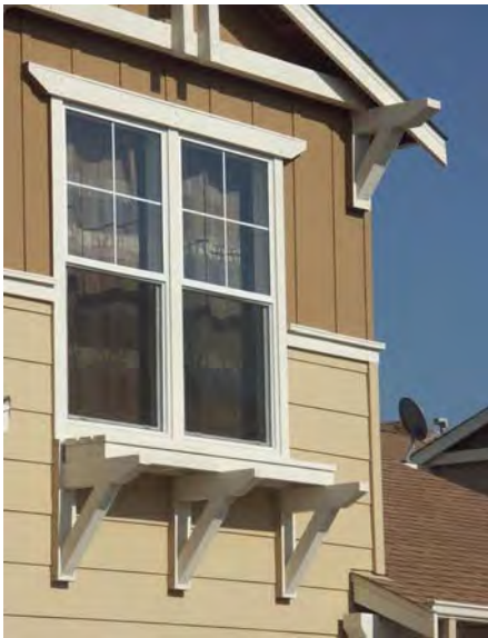
At shallow insets, projecting sills, molded surrounds, lintels and/or trim should be used to frame openings.
