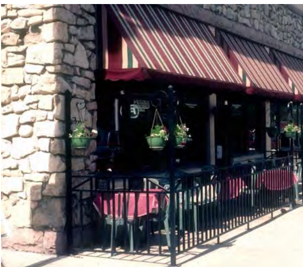
Stone veneer can be used as an accent material, as shown above.
