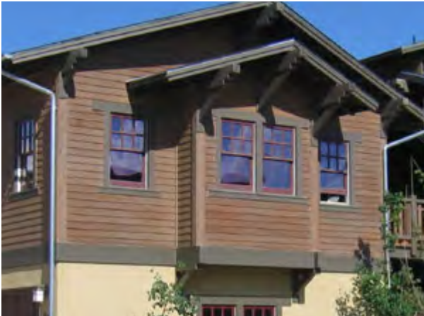
A Craftsman-style building with windows ganged together with a mullion separating the two windows.
