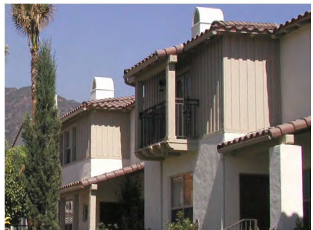
The vertical joints between the board and batten siding and stucco of this building occurs at the inside corner.
