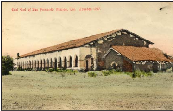
San Fernando Mission, San Fernando Valley History Digital Library, California State University, Northridge.
