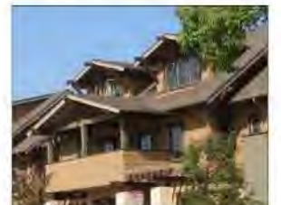
Upper floors are incorporated into the attic spaces and are lit by dormer windows.
