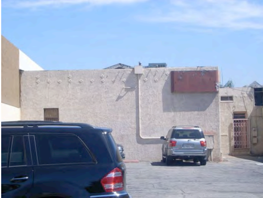
Celis Street near South Brand Boulevard: Partially-reinforced masonry building wall, deteriorated sign.
