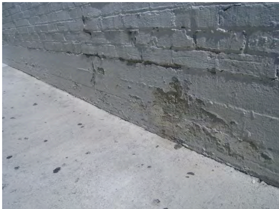
North Maclay Avenue and Truman Street: Close-up of cracked foundation.
