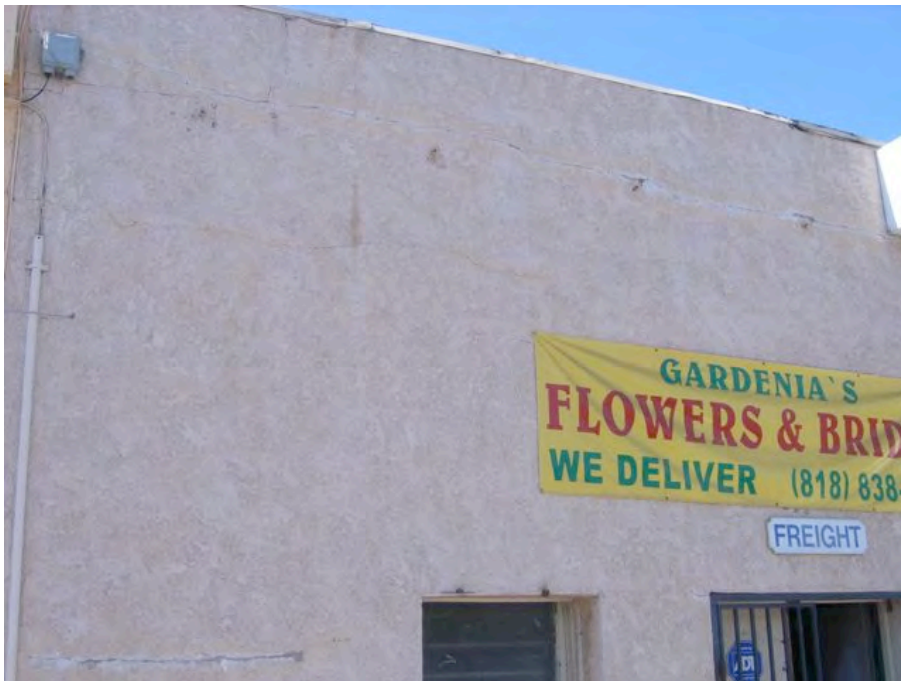
San Fernando Road near South Brand Boulevard: Cracks in reinforced masonry building wall with water damage and security bars.
