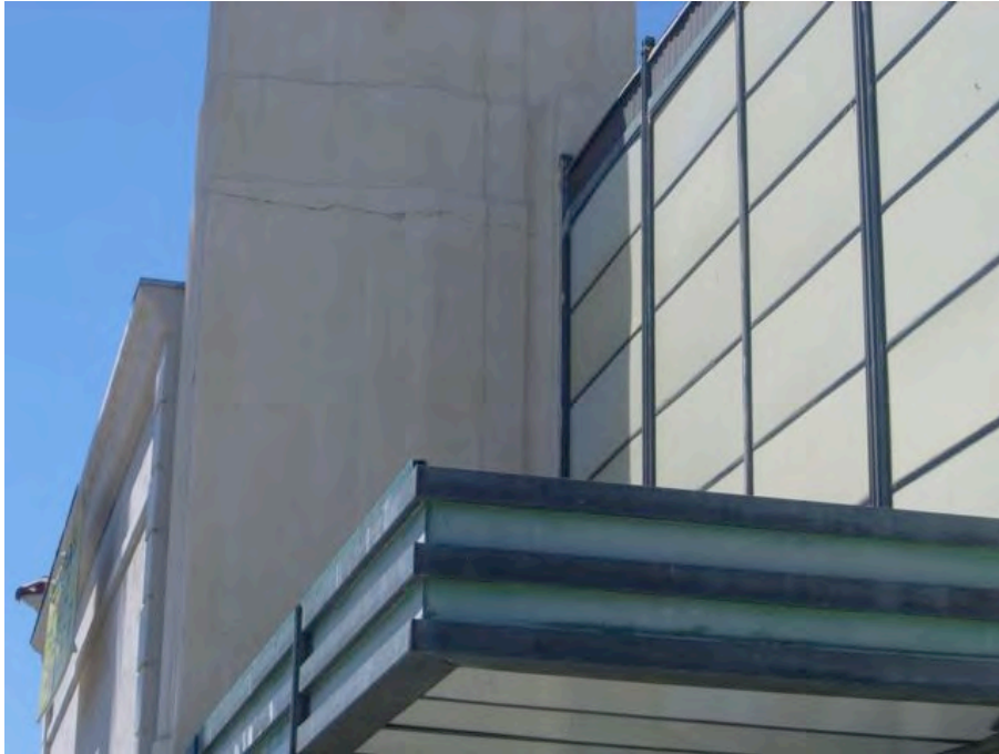
South Brand Boulevard near Pico Street: Cracks in stucco wall.
