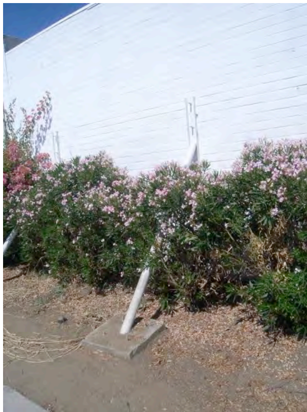
First Street near Orange Grove Avenue (rear): Brick wall reinforced with steel buttresses.
