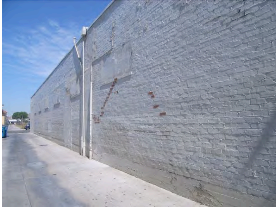
North Maclay Avenue and Truman Street: Reinforced brick building wall with cracks and peeling paint; cracked foundation.
