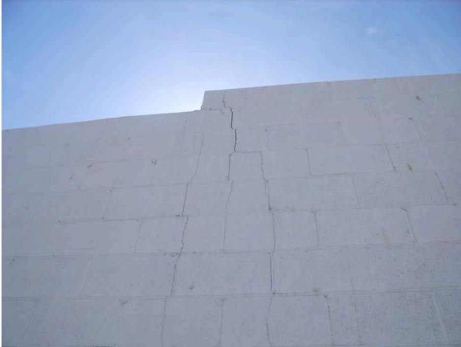
First Street near North Maclay Avenue: Extensive cracking in industrial building wall.
