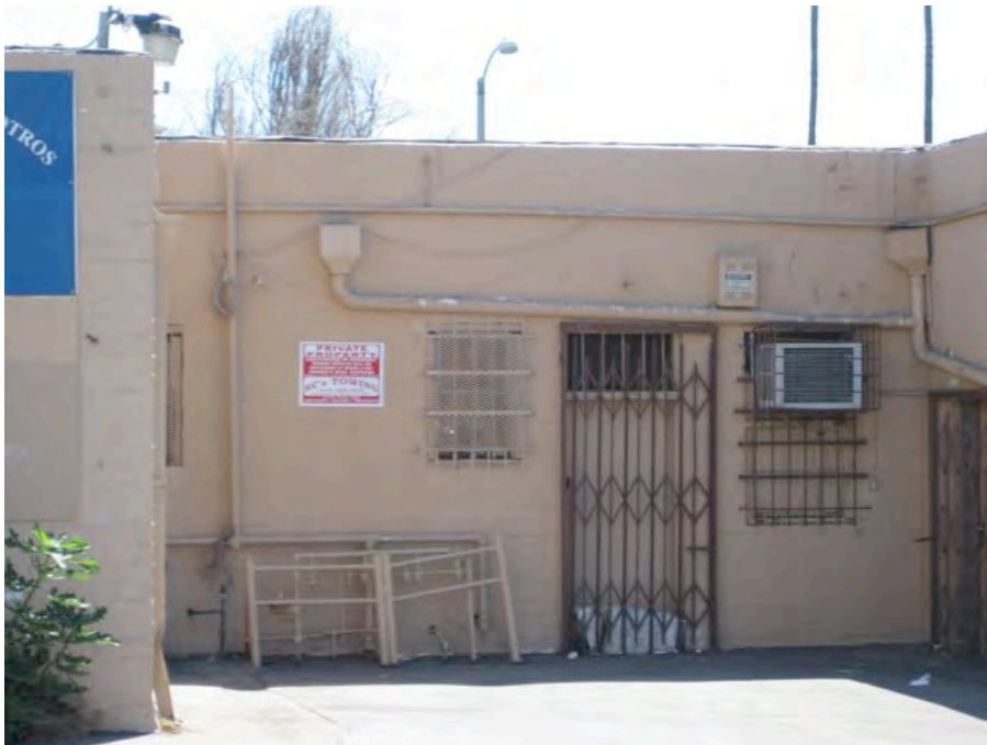
Celis Street near South Maclay Avenue: Unreinforced brick structure with exterior wiring and plumbing and security devices.
