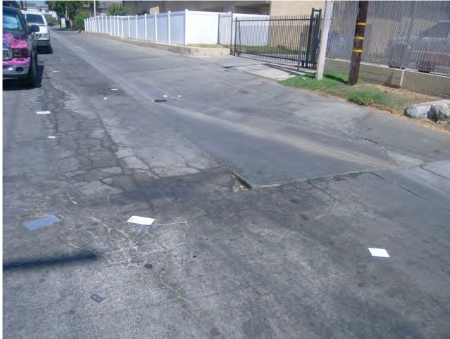
Orange Grove Avenue near First Street (rear): Deteriorated pavement, drainage to centerline of alley.
