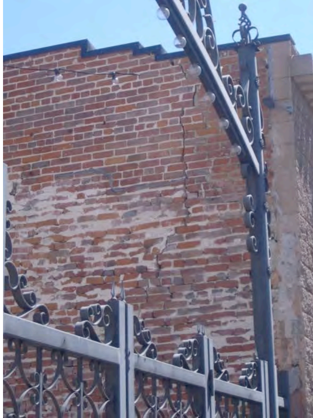
San Fernando Road near South Maclay Avenue, rear: Close-up of extensive cracking in brick wall.
