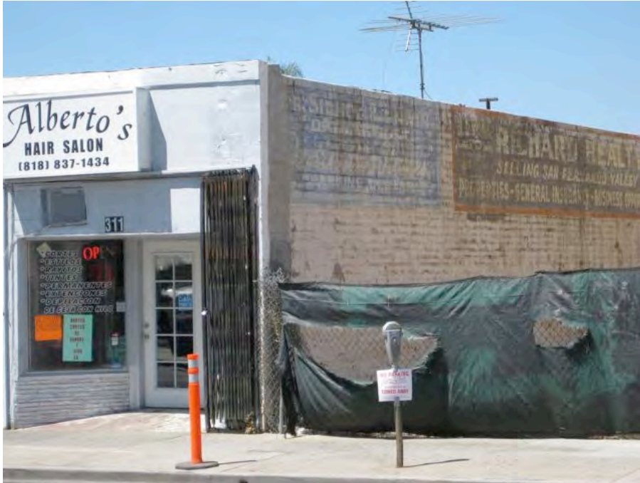
Celis Street near South Maclay Avenue: Unreinforced masonry building wall with peeling paint.
