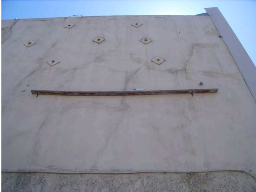
Celis Street near South Brand Boulevard: Close-up of extensive cracking and water damage in partially-reinforced concrete wall.
