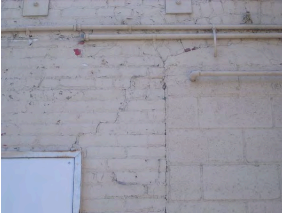
San Fernando Road near South Brand Boulevard: Close-up of cracks in reinforced brick wall, peeling paint.
