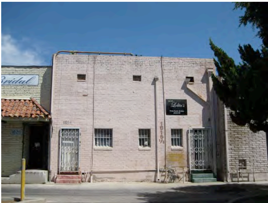
Celis Street near South Brand Boulevard: Cracks in unreinforced masonry building wall.
