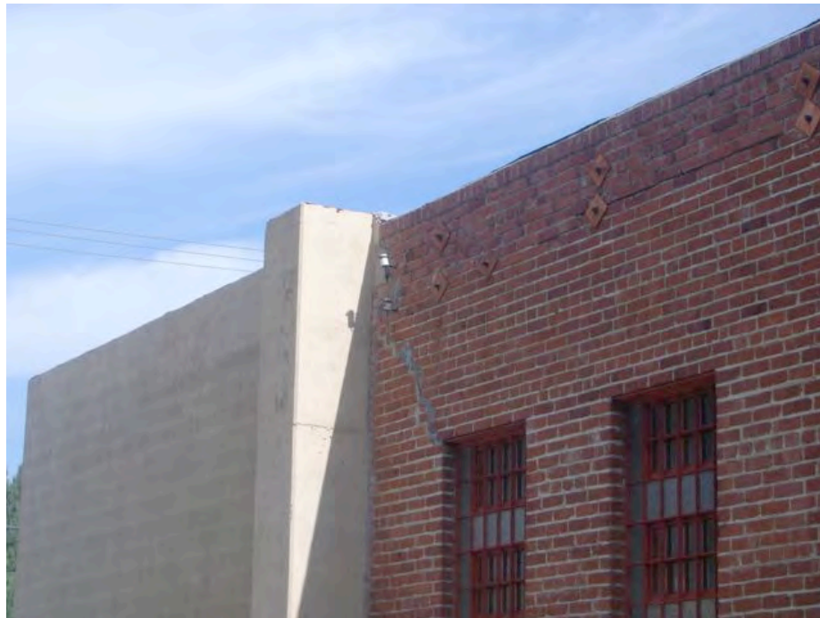
First Street near North Hagar Street: Patched cracks in partially reinforced brick building wall.
