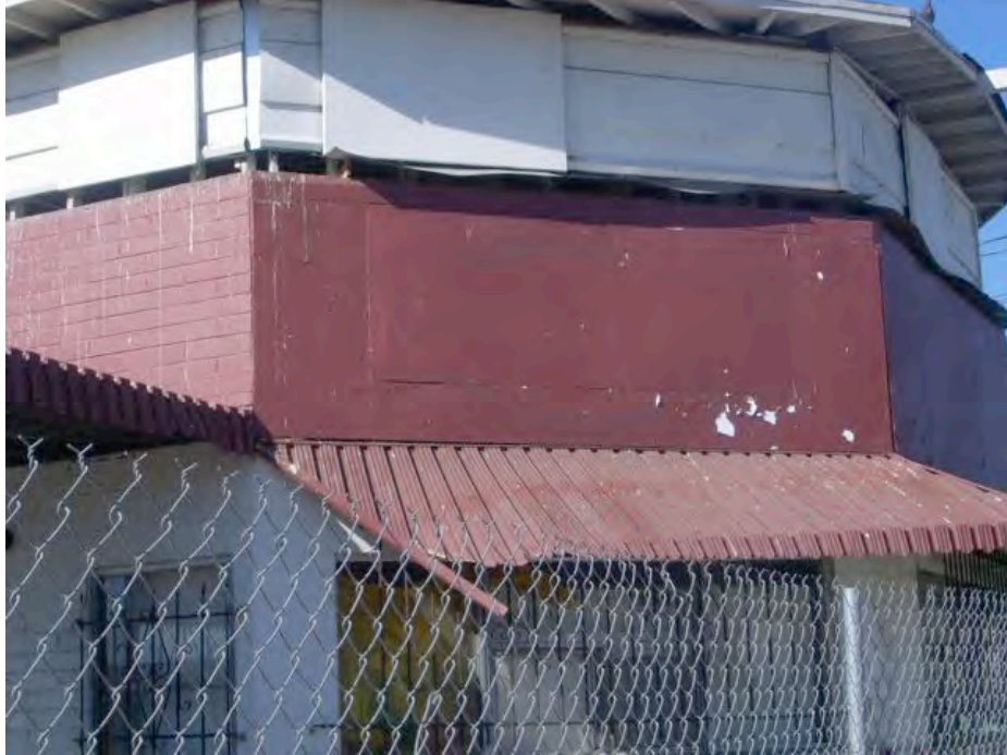
South Huntington Street near Truman Street: Close-up of deteriorating roofing, boarded windows, security grates, and peeling paint.
