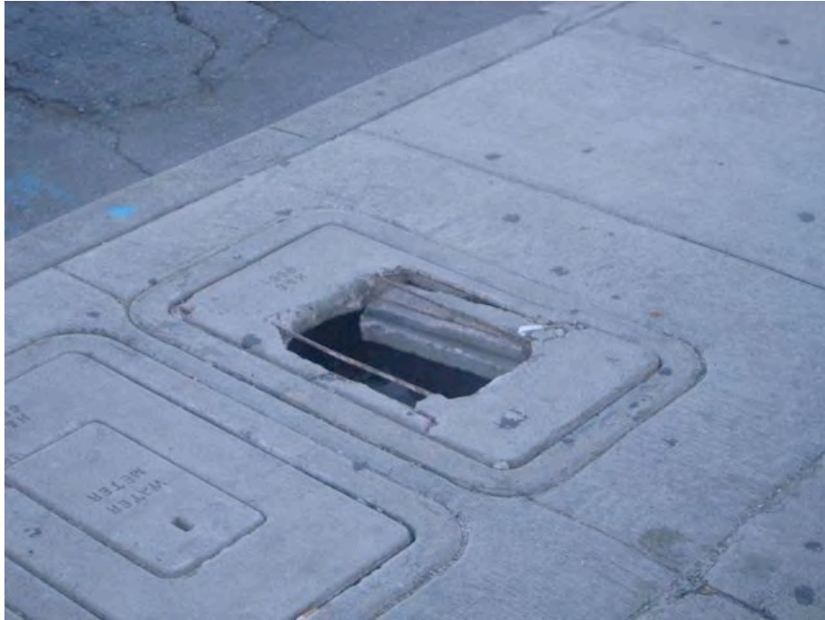
San Fernando Road near South Lazard Street: Damaged and sidewalk utility cover creating a hazardous condition for pedestrians.
