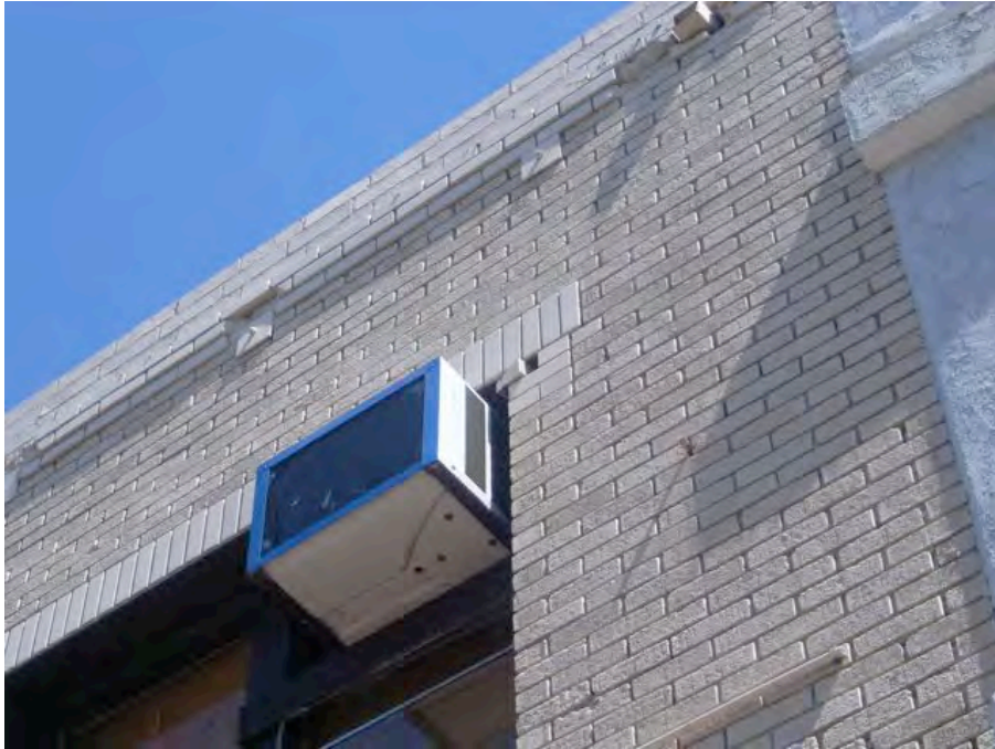
San Fernando Road near South Brand Boulevard: Reinforced brick building wall with cracks in wall and displaced bricks.
