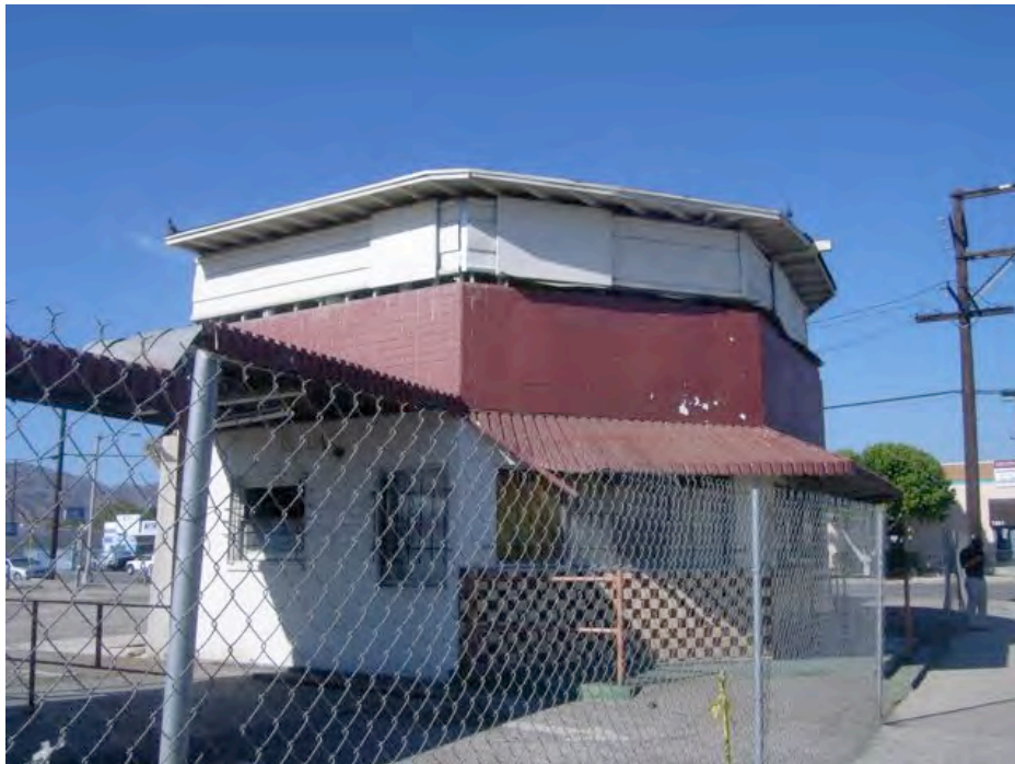
South Huntington Street near Truman Street: Vacant building with deteriorating roofing, boarded windows, security grates, peeling paint, and informal and substandard wall repairs.
