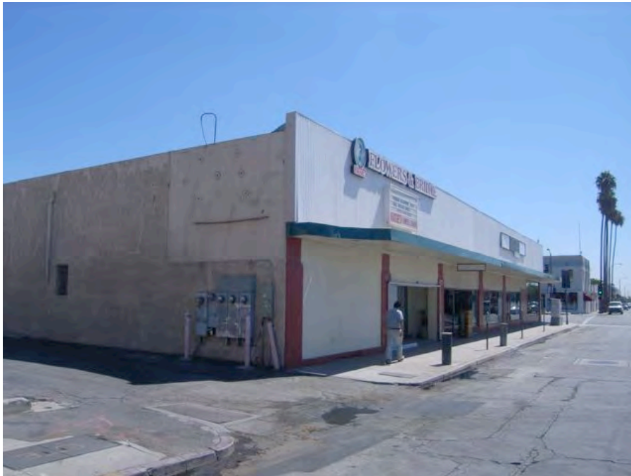
Celis Street near South Brand Boulevard: Extensive cracking in reinforced masonry building wall; deteriorated pavement and sidewalk.
