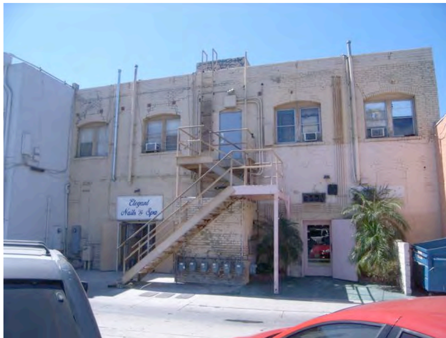
San Fernando Road near South Brand Boulevard (rear): Reinforced brick building with cracks in wall and peeling paint.
