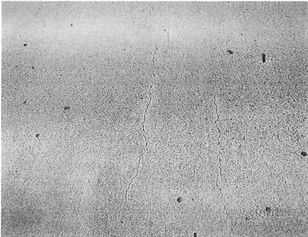
Photo 7 – Deck Cracks
