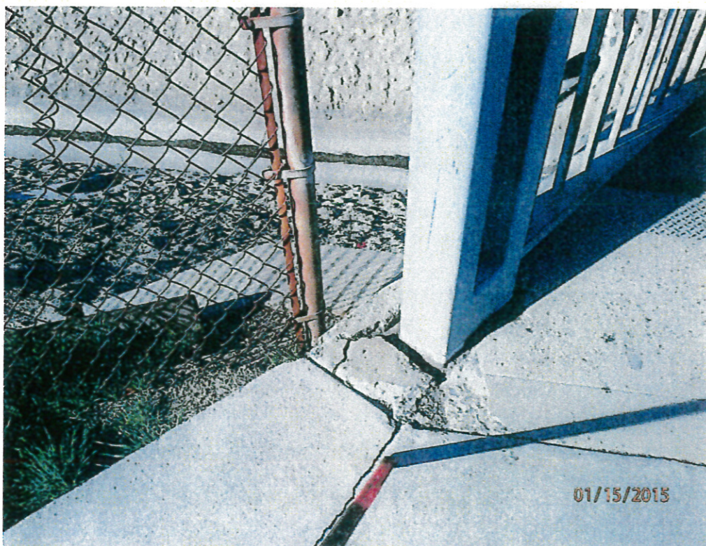
Photo 4 – Spalling at East End Post
