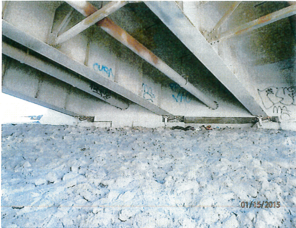
Photo 5 – Surface Rust on Girders and Bearings
