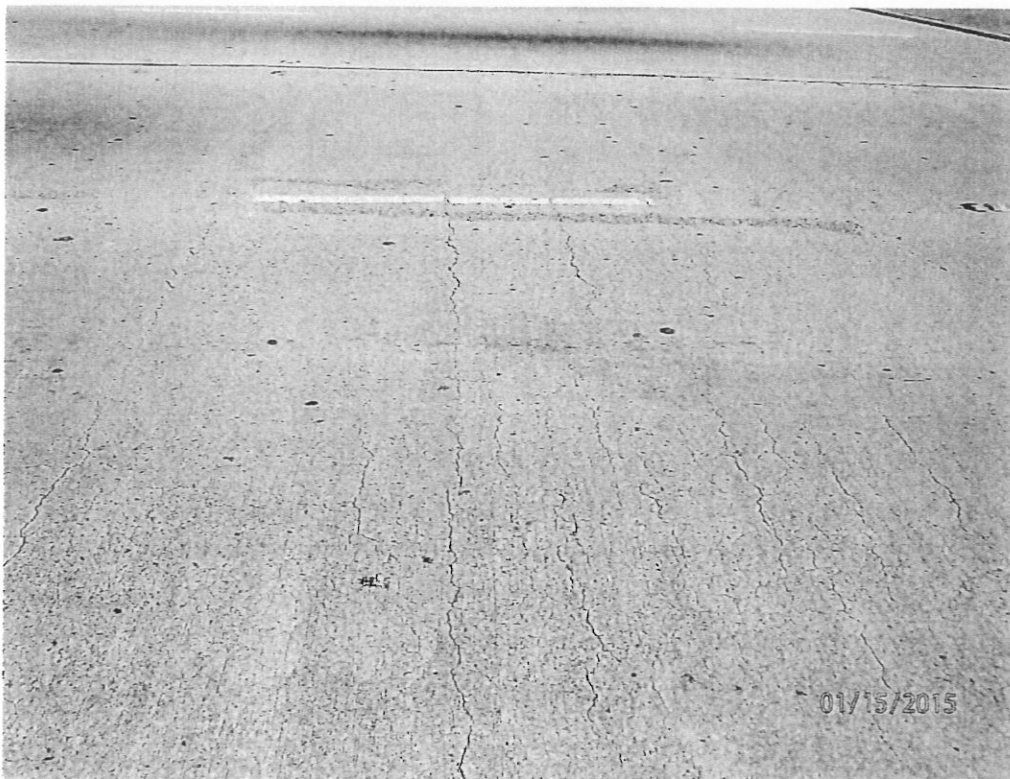
Photo 6 – Deck Cracks
