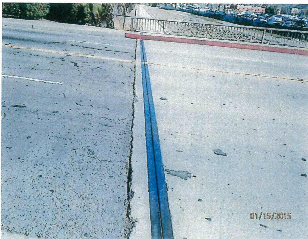
Photo 4 – West Open Joint
