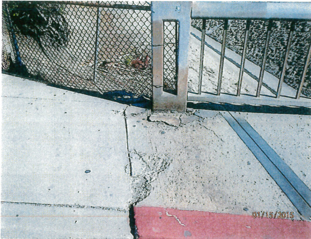
Photo 3 – Spall at End Post and Rusting Rails
