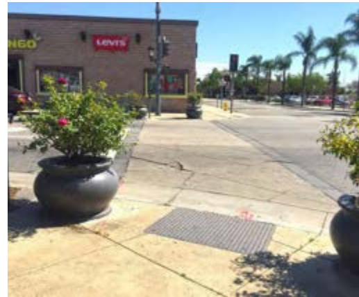
This crosswalk at Maclay Avenue and First Street has lost its markings over time, and could be difficult to see at night.
