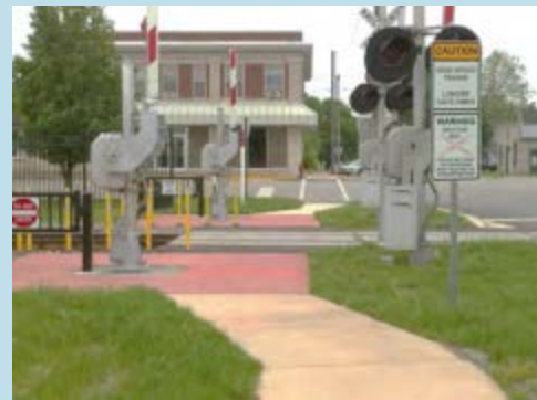
Railroad crossing with pedestrian supportive infrastructure (warning signs, continuous sidewalk, pedestrian gates, etc.)
