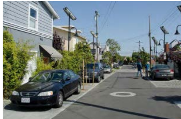
This street has removed curbs and uses textured pavement to visually narrow the street and invites people to walk down the middle.
