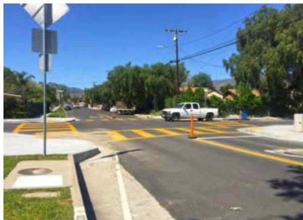
Curb extensions (curb pushed into the street in place of a parked car) shorten the crossing distance for people walking and can help slow cars down near the intersection, making it safer for everyone.
