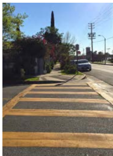
High-visibility crosswalks make crossings more obvious to drivers, and indicate the preferred crossing location to people walking. This is a ladder-style crosswalk; it's yellow because it is near a school.
