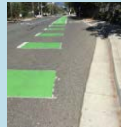
Colored bike lanes and conflict zone markings at intersection approaches encourage drivers to look for cyclists before changing lanes into a right-turn lane
