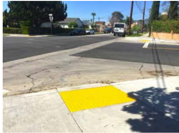
Diagonal curb ramps with truncated domes in San Fernando
