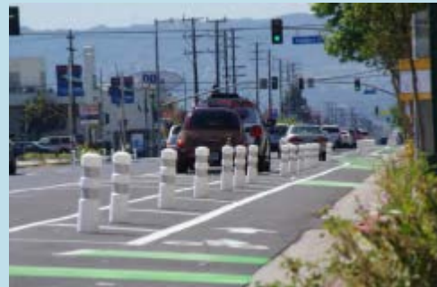
Protected bike lanes on Reseda Boulevard, with conflict points (merging lanes and driveways) painted green
