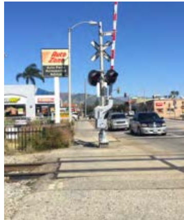
Pedestrian crossing at railroad tracks on Maclay Avenue. Currently, there are no signs, truncated domes, or gates warning walkers, and the sidewalk is rough across the tracks.
