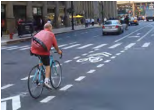
Bike Lane dashed marking through intersection
