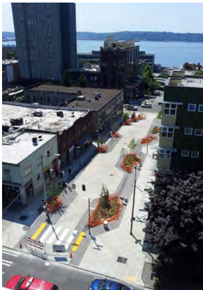
Bell Street, Seattle, shortly after shared street construction
