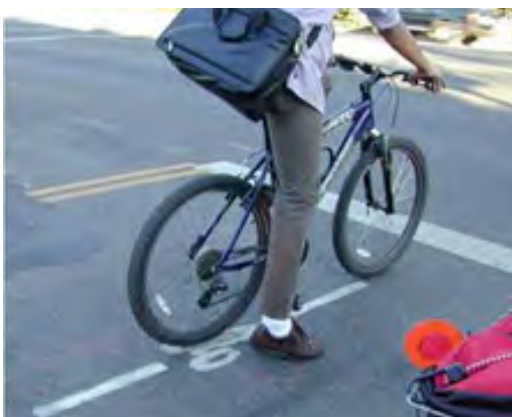
Cyclist Stopped to Activate Detector
