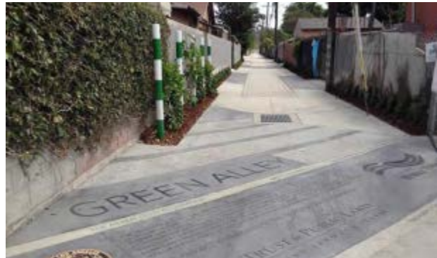
Green Alley built by Trust for Public Land in collaboration with City of Los Angeles that uses permeable surfaces to cool temperatures and collect water
