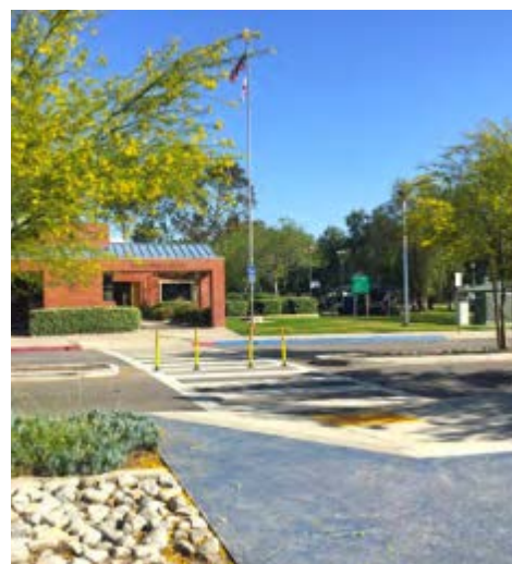
Uncontrolled crossing at Recreation Park (across Park Avenue) has been improved with large curb extensions (shortening the crossing distance), planted medians (provides refuge space for crossing pedestrians), and a high-visibility crosswalk marking.
