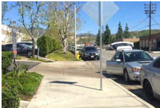
Missing sidewalk on route to Cesar Chavez Learning Academies (north of school)
