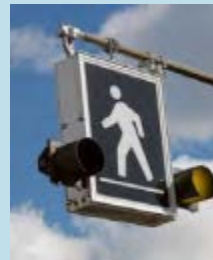
Overhead flashing beacon
