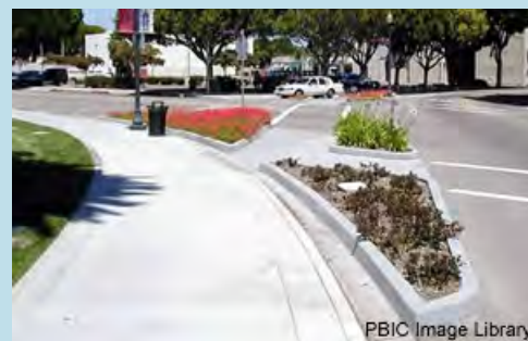
Islands used to reduce the curb radius and provide an area for landscaping (Credit: PBIC Image Library)
