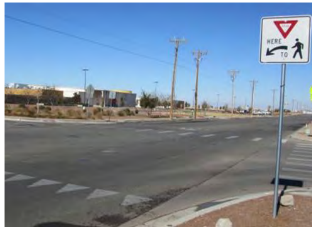
Advance Yield Markings & Sign at crosswalk (Lee Engineering, LLC)
