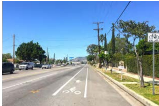
Bicycle lanes on Glenoaks Boulevard (east of Arroyo Ave) that end at the San Fernando border.
