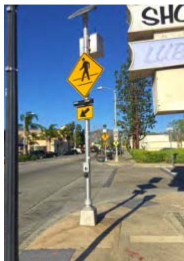
Pedestrian-activated Rectangular Rapid Flashing Beacon (RRFB) at an uncontrolled crossing on Maclay Avenue. When the button is pushed, two bright LED lights flash back and forth, signaling to oncoming drivers that someone is trying to cross the street.
