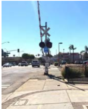
Pedestrian crossing at railroad tracks on Maclay Avenue. Currently, there are no signs, truncated domes, or gates warning walkers, and the sidewalk is rough across the tracks.
