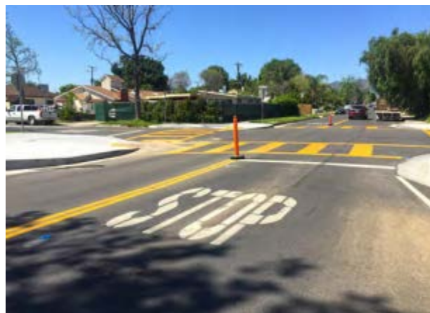
Advanced stop bars (bar behind crosswalk, in front of STOP pavement legend) show drivers where to stop, and help prevent cars from encroaching into the crosswalk. San Fernando has installed curb extensions and upgraded pavement markings throughout the city
