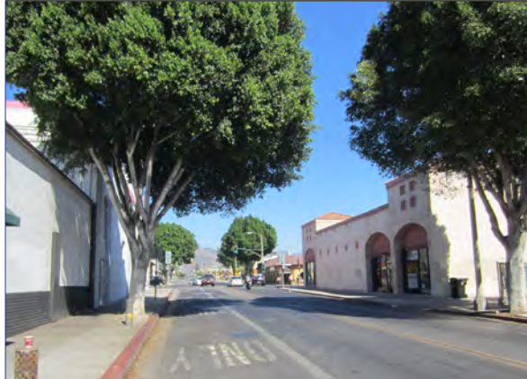
FIG. 11: EXISTING CONDITION SOUTH OF SAN FERNANDO RD.
