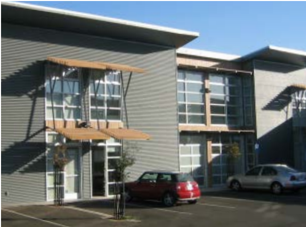
Canopy made of wooden slats on their sides providing shade but not protection from rain
