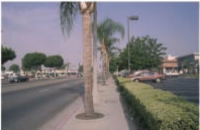
Existing view looking west along Truman Street
