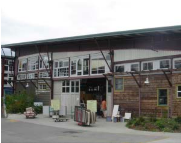
The facade of this industrial buildings incorporates the products that are sold within: doors and windows of different sizes and shapes.
