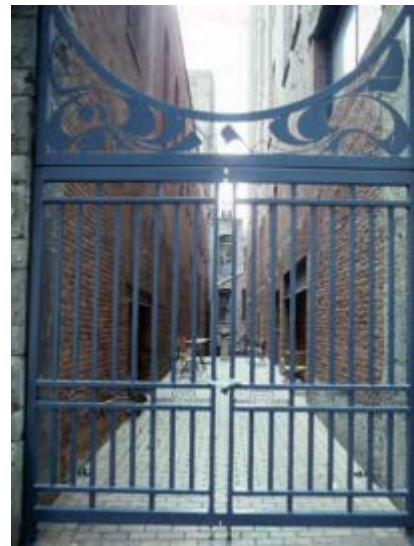
Wrought and painted iron as fence materials.
