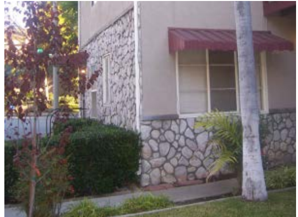
AVOID: Stone veneer that does not wrap the corner gives away the fact that is an applied veneer.
