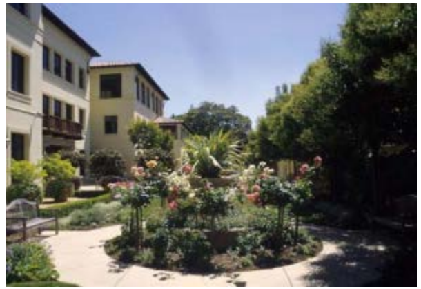
A common courtyard for residential units.
