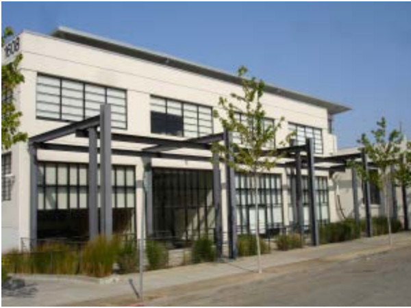
A contemporary building with skeleton frame canopy.
